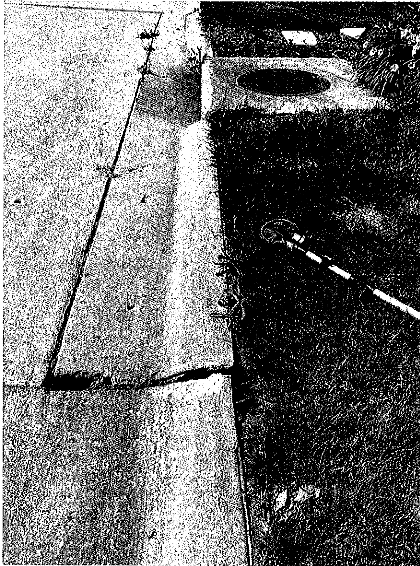
Line 1, fill apron void. crack fill around as well.
